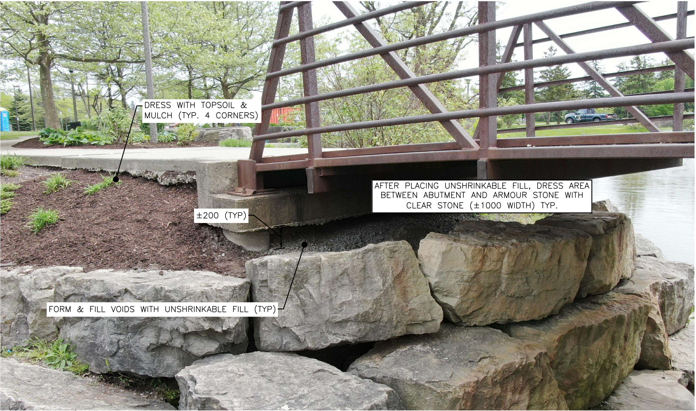
PHOTO #1 – EAST ABUTMENT (WEST ABUTMENT SIMILAR)
