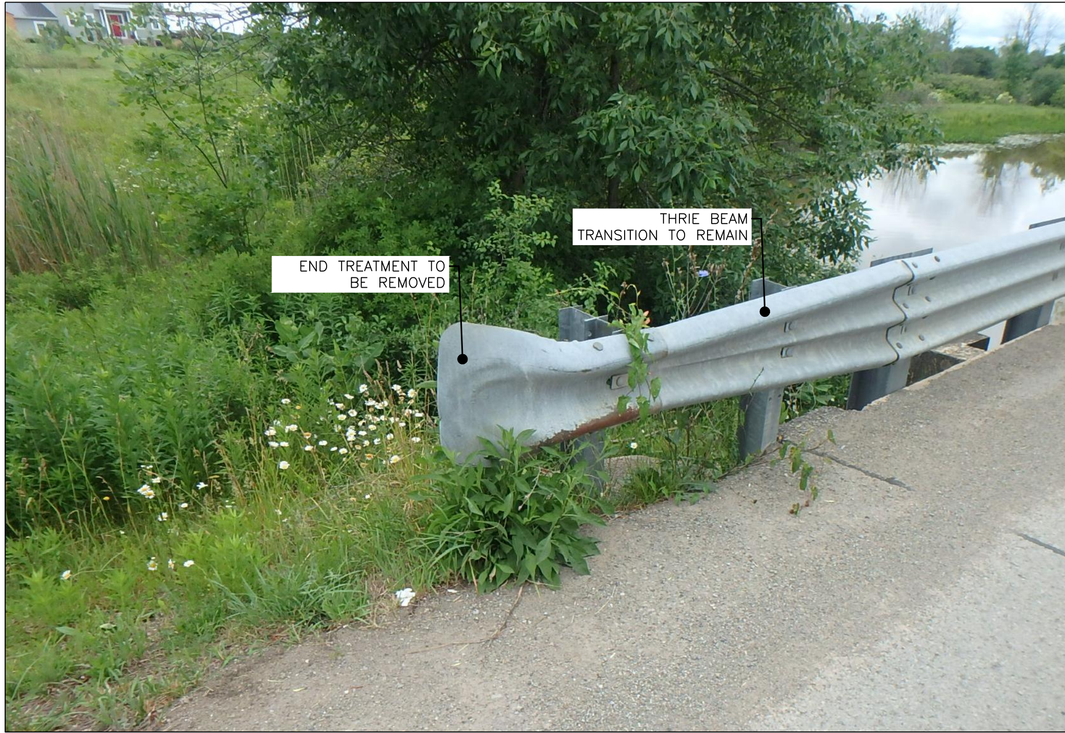
PHOTO #1 – EXISTING SOUTH EAST GUIDERAIL
