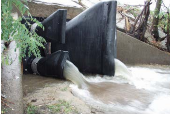
Figure 7.1 Backflow Prevention Example (Red Valve Company, Inc. 2020)
