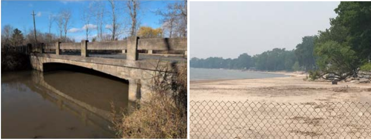
Figure 4.10 Thunder Bay Road Bridge (left) and Lake Erie Shoreline (right)
