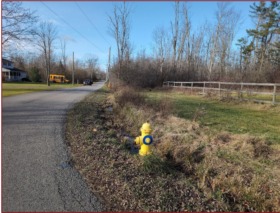
Image 12: Ditch and Culvert Along Shirley Road
