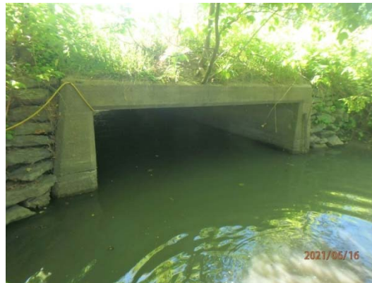
Above: Existing Concrete Rigid Frame Culvert at Black Creek Road (north end).
