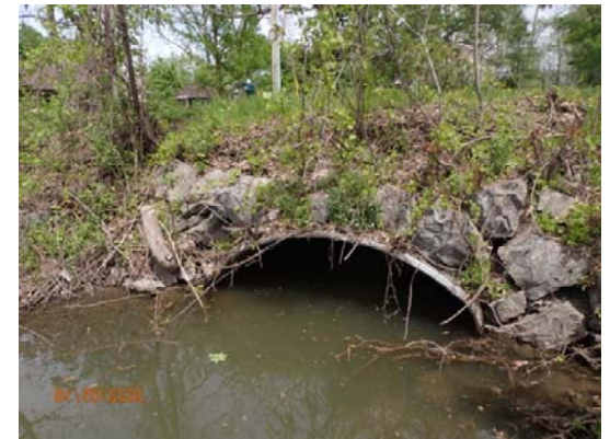
Above: Existing Corrugated Steel Pipe Culvert at Black Creek Road (south end).
